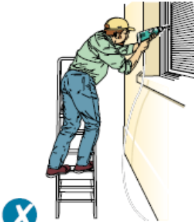
Figure 2a Incorrect - steps side-on to work activity
