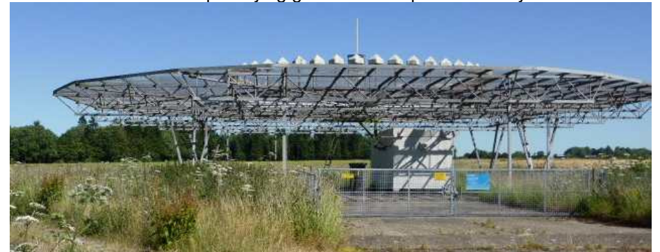
Doppler VHF Omni-range radio beacon marking the centreline of the airway to and from Heathrow.
